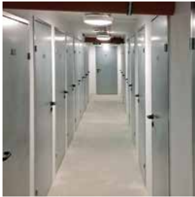
RESIDENTIAL ESTATE UNIVERSAL DOORS TO UTILITY ROOMS
